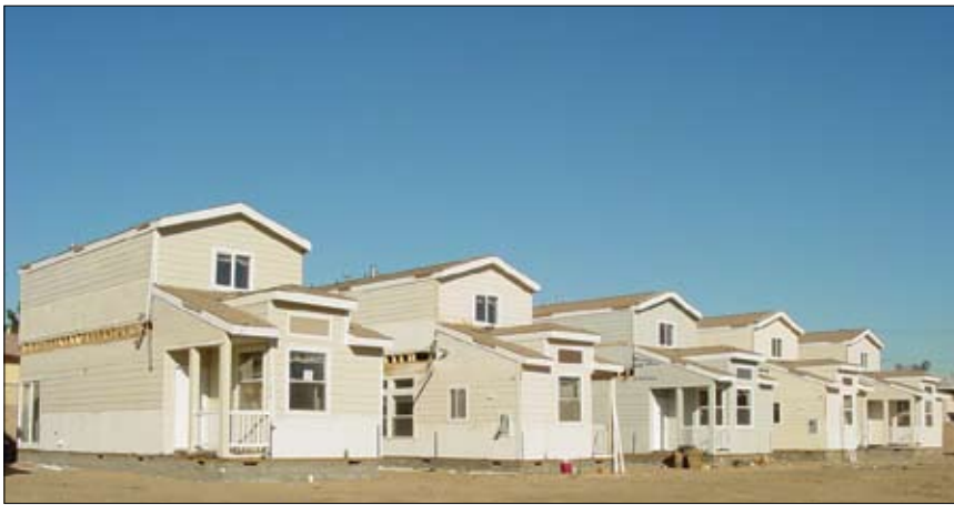
Home delivery and installation in process...
