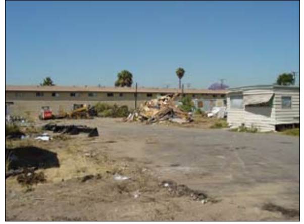
Demolition and the Renaissance begins!
